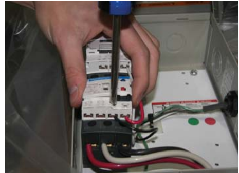
PICTURE 4: Disconnecting Relay Wires
