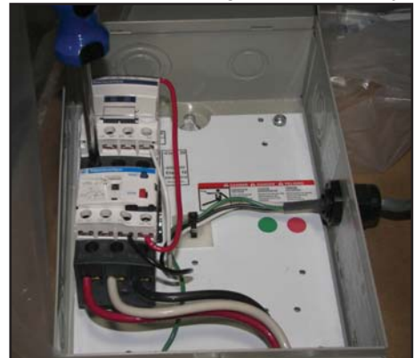
PICTURE 4: Disconnecting Relay Wires
