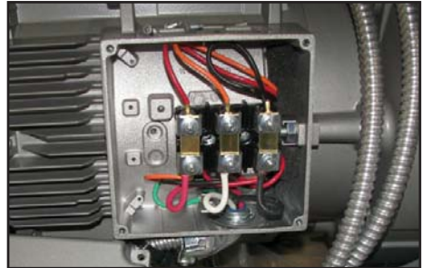
PICTURE 2: 440V Becker Pump Wiring
