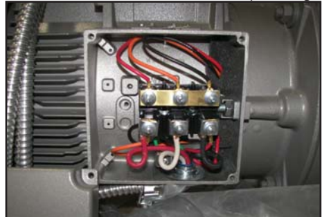
PICTURE 3: Detaching the Overload Relay
