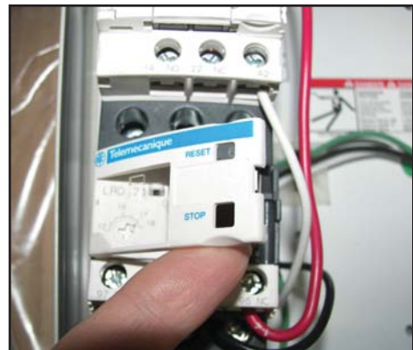
PICTURE 7: Accessing Amperage Dial Settings
